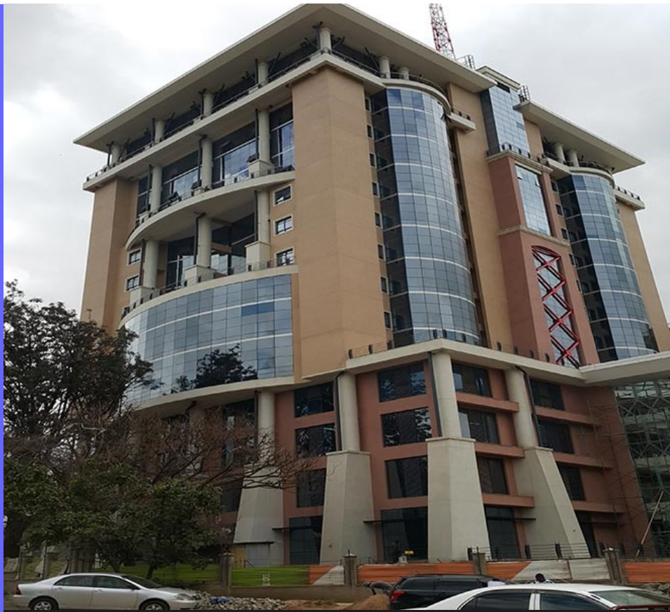
A sample of some of our works: REAL INSURANCE OFFICE BLOCK, NAIROBI
